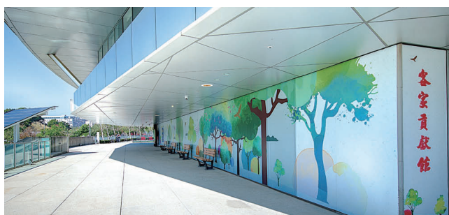
行政區三樓戶外平臺 Square in front of 3F, Administration Offices
